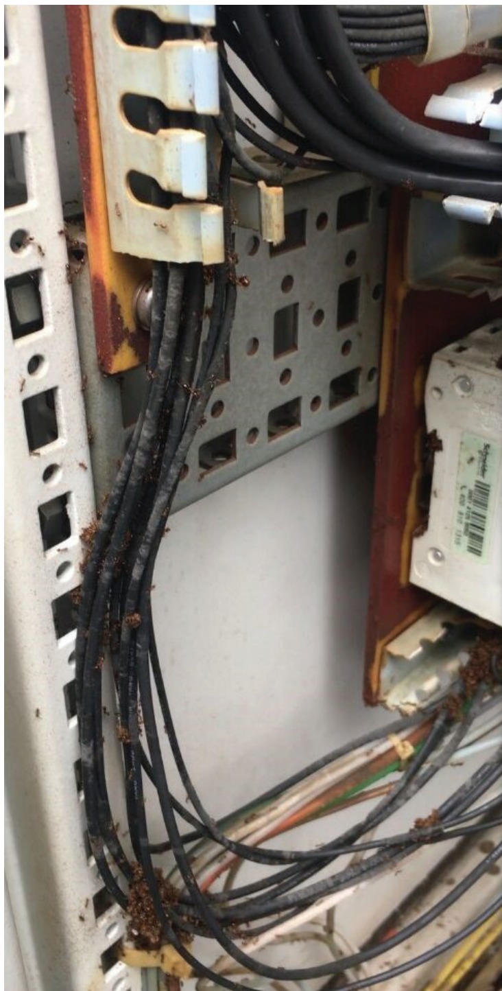
Figure 7. Solenopsis invicta workers attack a cable box (photo provided by Guangzhou Metro Group Co., Ltd).
